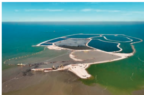
Figure 3: Overview of the Island construction works (Source Boskalis)
