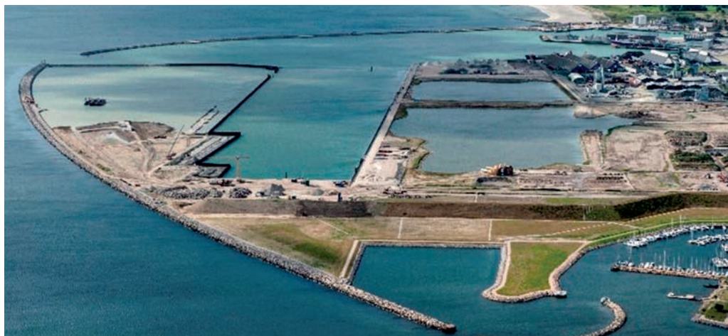
Uniterminal | Port of Koege | Denmark (2016). 4 000 t of AMLoCor © steel sheet piles installed.
