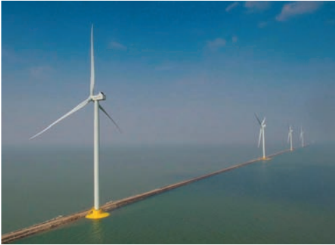
Figura 6: Deep (left) and gravity (right) foundation integrated in a rubble mound breakwater in Nangang WF (left, Source: Siemens-GAMESA) and Port of Gijon (right).
