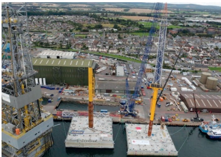
Figure 5: Meteorological Masts of Inch Cape and Moray Firth built over caisson-type solution.
